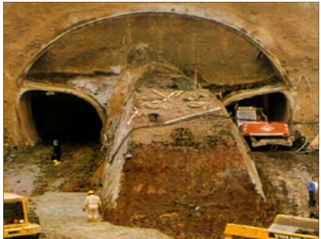
SEM Operation at a Tunnel Portal 2
