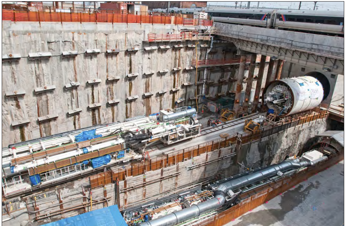
Mixed-Face TBM 2
